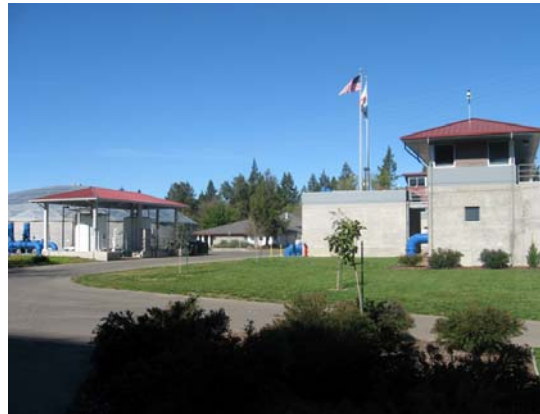
The City of West Sacramento's Bryte Bend WTP. One of the surveillance cameras located at the plant is visible on the building to the right.
